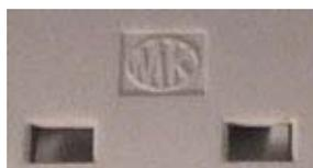
If your sockets are the type in which the shutters are operated by the insertion of both the lower pins at the same time, like this MK model, the closed shutters will look something like this. You can see that the shutters are shaped to ensure they operate only if a plug is inserted.
